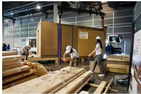
Workers assemble modular timber components in the Industrialised Construction Hall at FIMMA + Maderalia, where new exhibitors including Egoín, Bariperfil, Cadwork, Thermochip and others will showcase solutions for industrialised and sustainable building from 10–13 November at Feria Valencia. Image: Feria Valencia
