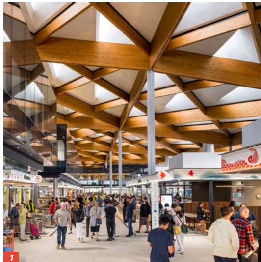
1/ View of the internal timber roof structure showing the wave light panels.
