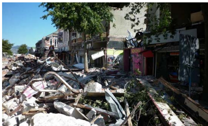
Christchurch's Colombo Street after the 2011 earthquake. The city's masonry buildings were particularly hard hit. Image: CC/Schwede66
