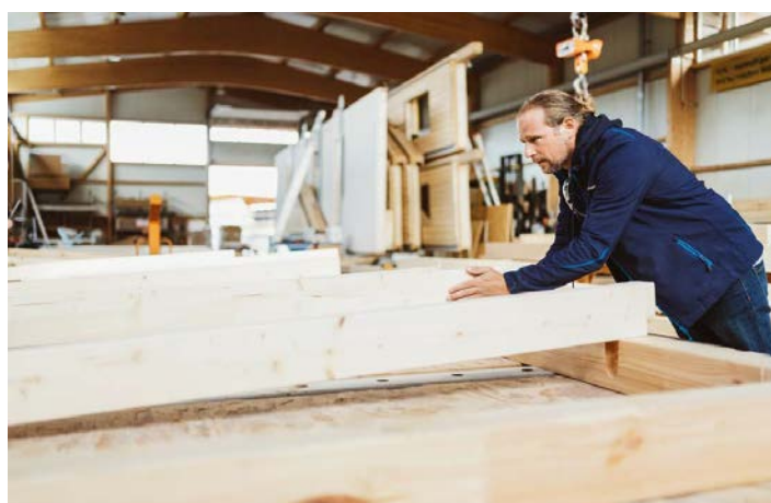
Prefabricated timber housing allows for faster, more efficient construction in offsite facilities that lower risks to workers and to weather exposure. Image: Shutterstock/stockfour
