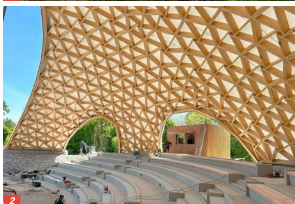
1/ The completed Parkarena in Furth im Wald, a sustainable timber venue with its lightweight PVC membrane roof and double-curved elegance, serving as a lasting community hub. 2/ The Parkarena's intricate honeycomb-like timber gridshell during construction, showcasing the reciprocal geometry of straight glulam beams and the emerging stage and seating that blend with the natural surroundings. Images: str.ucture GmbH
