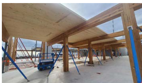
Australian mass timber, such as these CLT roof and floor panels by NeXTimber at the Flinders University Factory of the Future and Tonsley Technical College project, will help us meet carbon targets. Photo: courtesy NeXTimber
