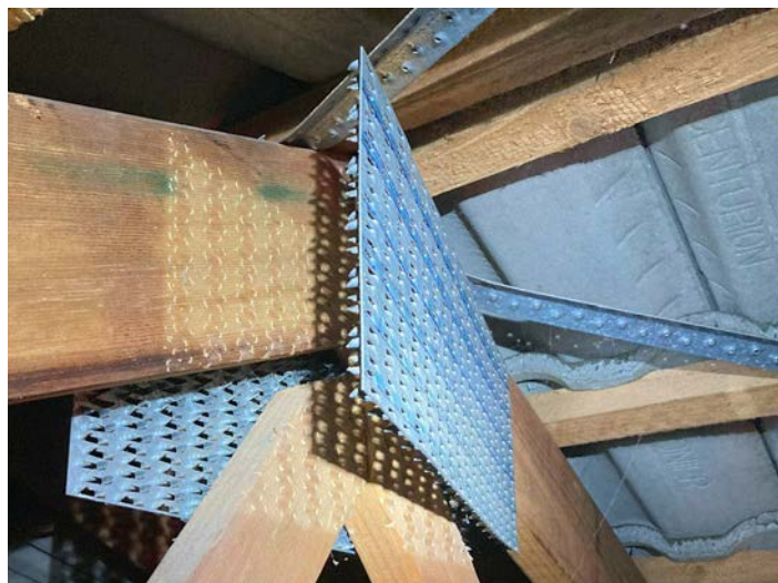
A large plate failure caused by incomplete pressing. All photos: Paul Davis
