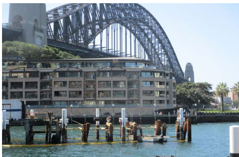
Structural timbers and some of the piles at Campbells Cove are being replaced with the turpentine find. Photo: supplied
