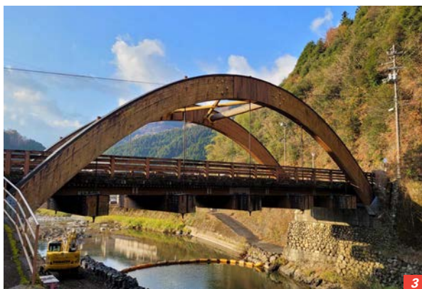
3 & 4/ Vehicle timber bridges in Japan (left) and Norway. Photos: courtesy Dr Gary Raftery
