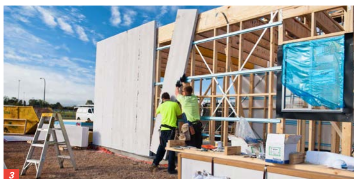
1, 2 & 3/ Prefabricated wall segments are installed on a house project. Images: Big River Group
