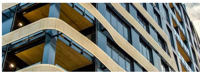
Monterey Apartments in Brisbane, a hybrid concrete, CLT and glulam residential tower delivered by Aurecon. Image: courtesy Aurecon Group
