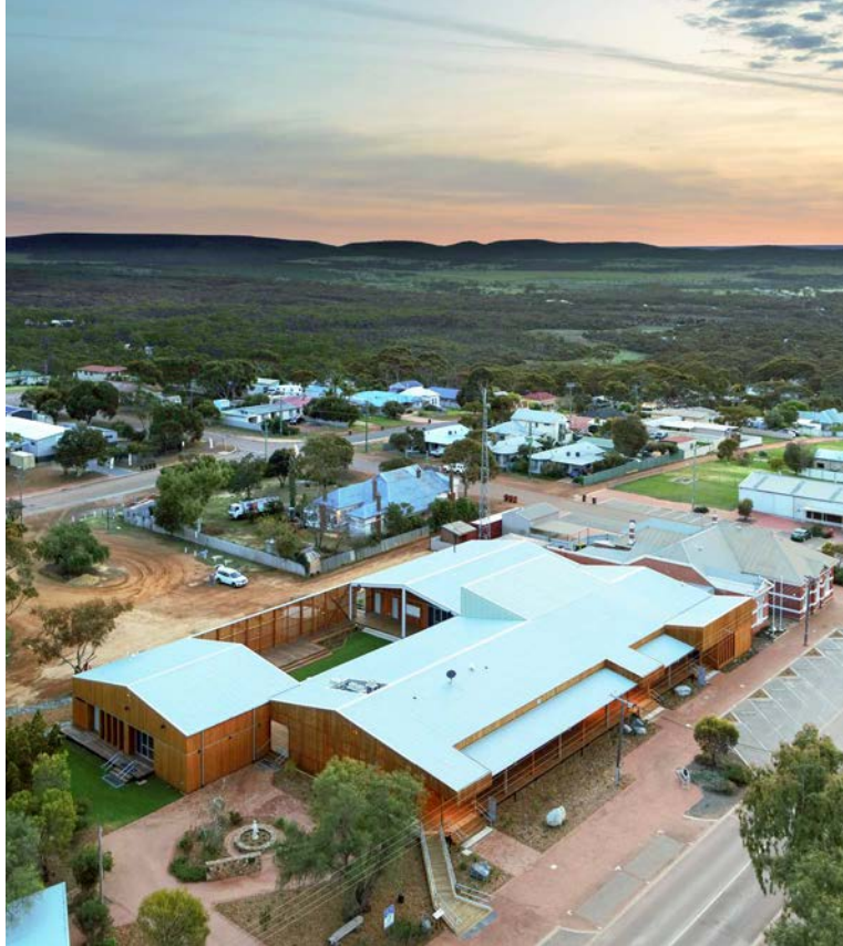
The gleaming set of buildings has become the heart of the local community. Photo: Johnathan Trask - courtesy ATC and Peter Hobbs Architecture
