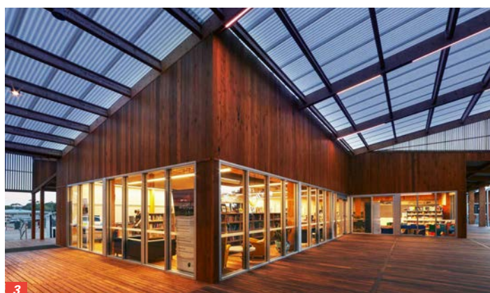
1/ Floating on concrete piers, the building is both accessible and movable. Photo: Johnathan Trask - courtesy ATC and Peter Hobbs Architecture
