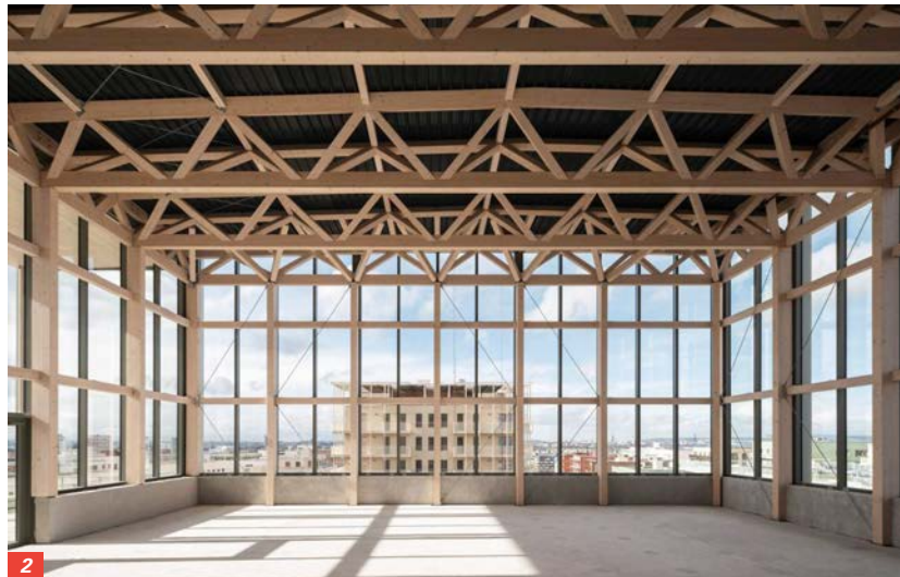
1/ The striking building in the Paris Olympic villages features mass timber, exposed beams and terracotta tiles.
