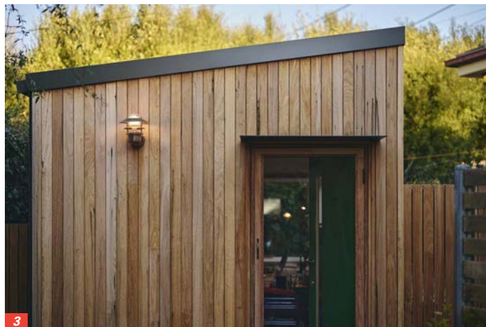
1/ Hackett Gardens House built with recycled cladding, decking, posts and beams, and re-milled flooring.
