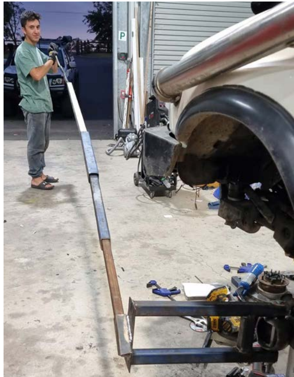
Learning a valuable lesson on lateral torsional buckling!
