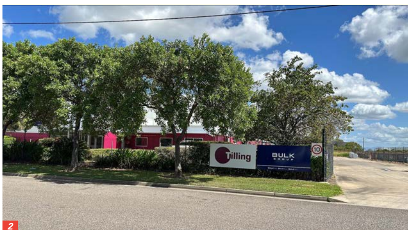
1/ The racks are filling up at Tilling Townsville, ready for the grand opening in a fortnight. 2/ The new facility has ample truck and ute space, wide racking for easy order picking and a central Townsville location.
