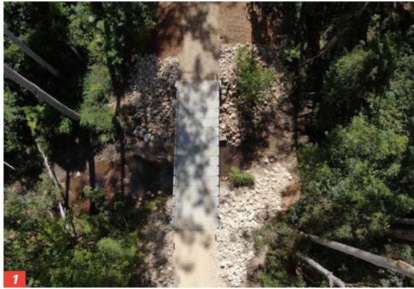
1/ Blackbutt Road bridge has now been fully completed.
