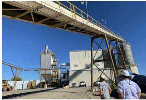
Wellons 15MWt with 1.5MWe Energy System.
