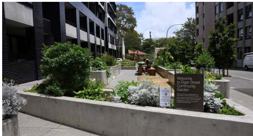
The new Elger St housing in Sydney's Glebe delivered 158 social dwellings. Photo: Sardaka, CC BY-SA 4.0, via Wikimedia Commons
