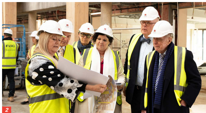
1/ The newly completed building is full of light and open spaces for collaborative work. Photos: courtesy Xcel Carpentry and Construction 2/ Juliette Churchill, executive director, property services at Macquarie University (far left), takes distinguished guests including the Hon. Michael Kirby (far right) through the plans for the Michael Kirby Law School Building last July. Photo: Macquarie University
