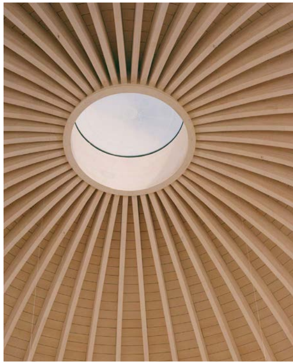
Glulam ribs lift a dome above the square room of the main temple, with light streaming in from both the top lantern and clerestory windows. Photo: Rory Gardiner
