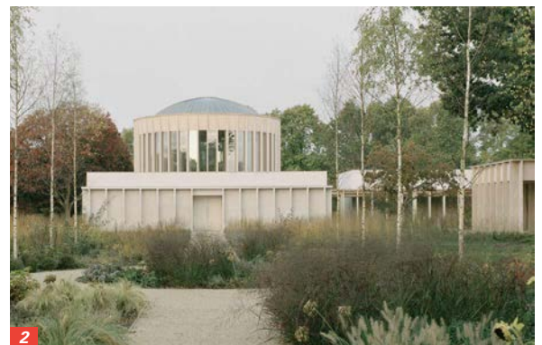
1/ The timber framing is visually expressed in multiple parts of the complex; digital scanning made sure the glulam used was all knot-free and consistent. Image: Rory Gardiner
