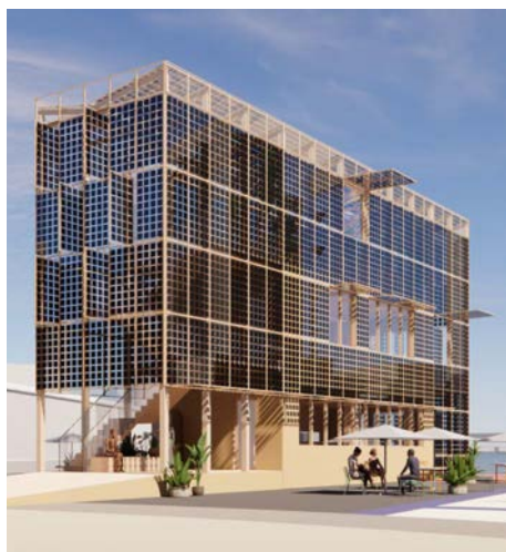
Timber construction and wood fibre insulation will make the Plus Prototype light and comfortable to live and work in.
