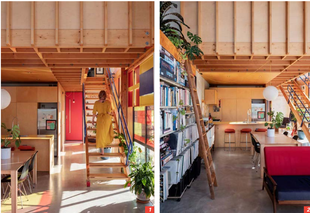
1/ Dowie Rose House has a concrete ground floor and back wall to soundproof against the adjacent railway and provide thermal mass, then glulam timber upper storey. Image: Sam Hartnett.
