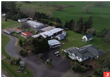
1 & 2/ Trainworld under construction. The designer-builder is Pierre Vuilleumier. 3/ Aerial view of the Timber Museum site, taken August 2023.
