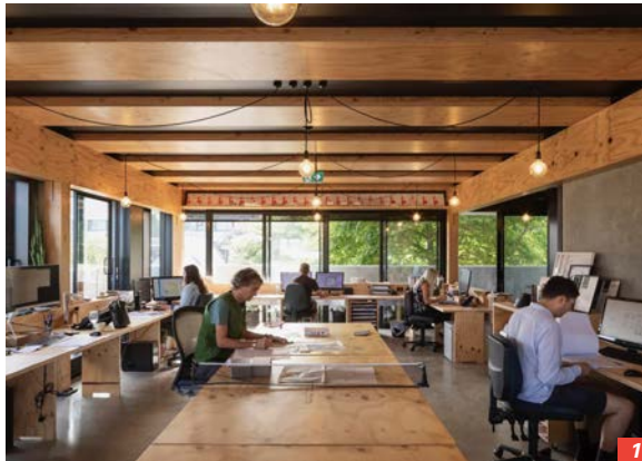
1/ Wall-E, winner of the Hybrid Building Award: notable for its fully expressed LVL post, beam and POTIUS floor elements. Image: Patrick Reynolds 2/ Tomohai ki Ahipara (cultural gateway to Ahipara, Northland): winner of the People's Choice Award. Image: BJ Natanahira
