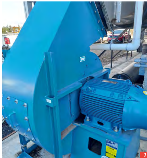
1/ The Brady blower - GMT's aeration valves controlled by WebMacs determine volume of airflow to each composting zone.
