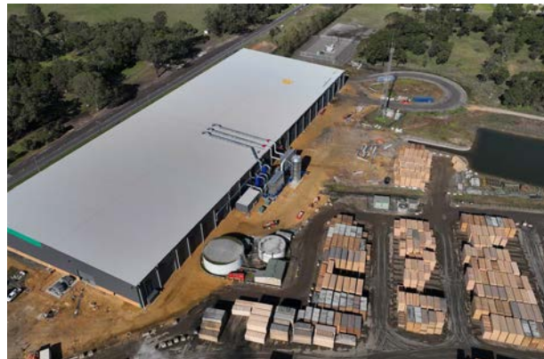
The NeXTimber facility is co-located at Timberlink's Tarpeena, SA, manufacturing facility.
