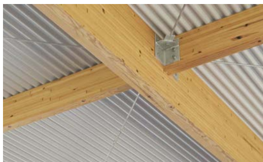
Glulam and tin reference classic Queensland construction materials.
