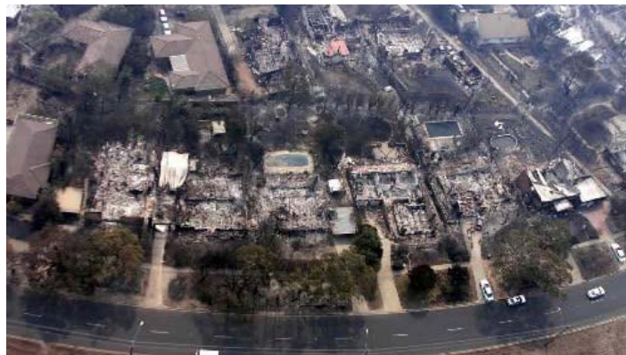
Homes in Canberra destroyed by bushfire reminds all of the importance of bushfire readiness. Photo: CBR ACT
