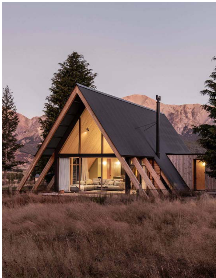
Adventure Whare: utilises “renewably grown and locally fabricated PLT mass timber panels”. Photo: Stephen Goodenough
