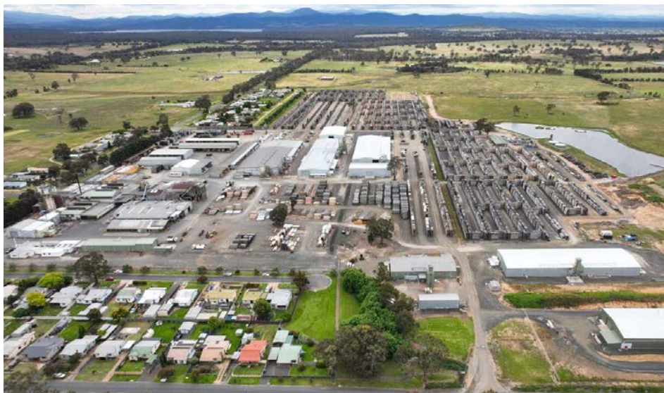
Australian Sustainable Hardwoods (ASH) sawmill and manufacturing facility, Heyfield, Victoria.
