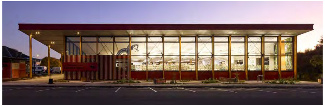
Motueka Public Library features locally sourced and fabricated timber elements. Photo: Jason Mann
