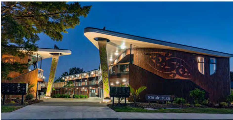
Auckland social housing project features CLT walls/mid-floors, resulting in reduced construction time.
