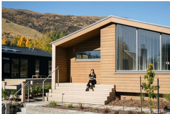
Timber, wool and double glazing ensure durable comfort in harsh conditions.
