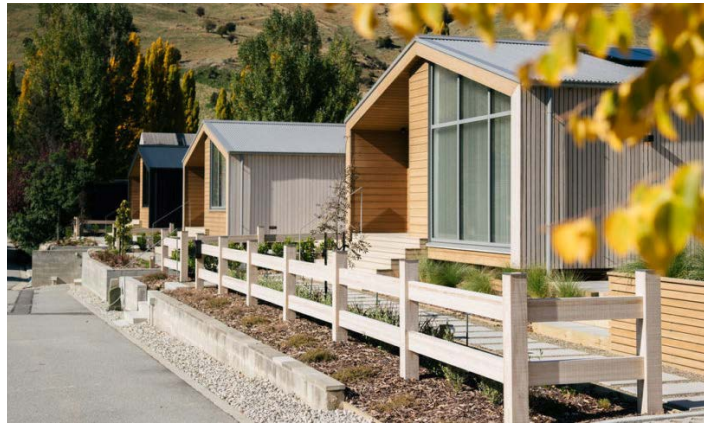
The villas were prefabricated in Christchurch and trucked to site.
