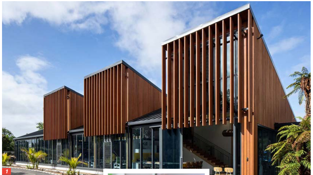
1/ Auckland Zoo administration building... timber highlights include the exterior fins, glulam portal frames, the mezzanine floors and decorative plywood linings. Photo: Simon Devitt.
